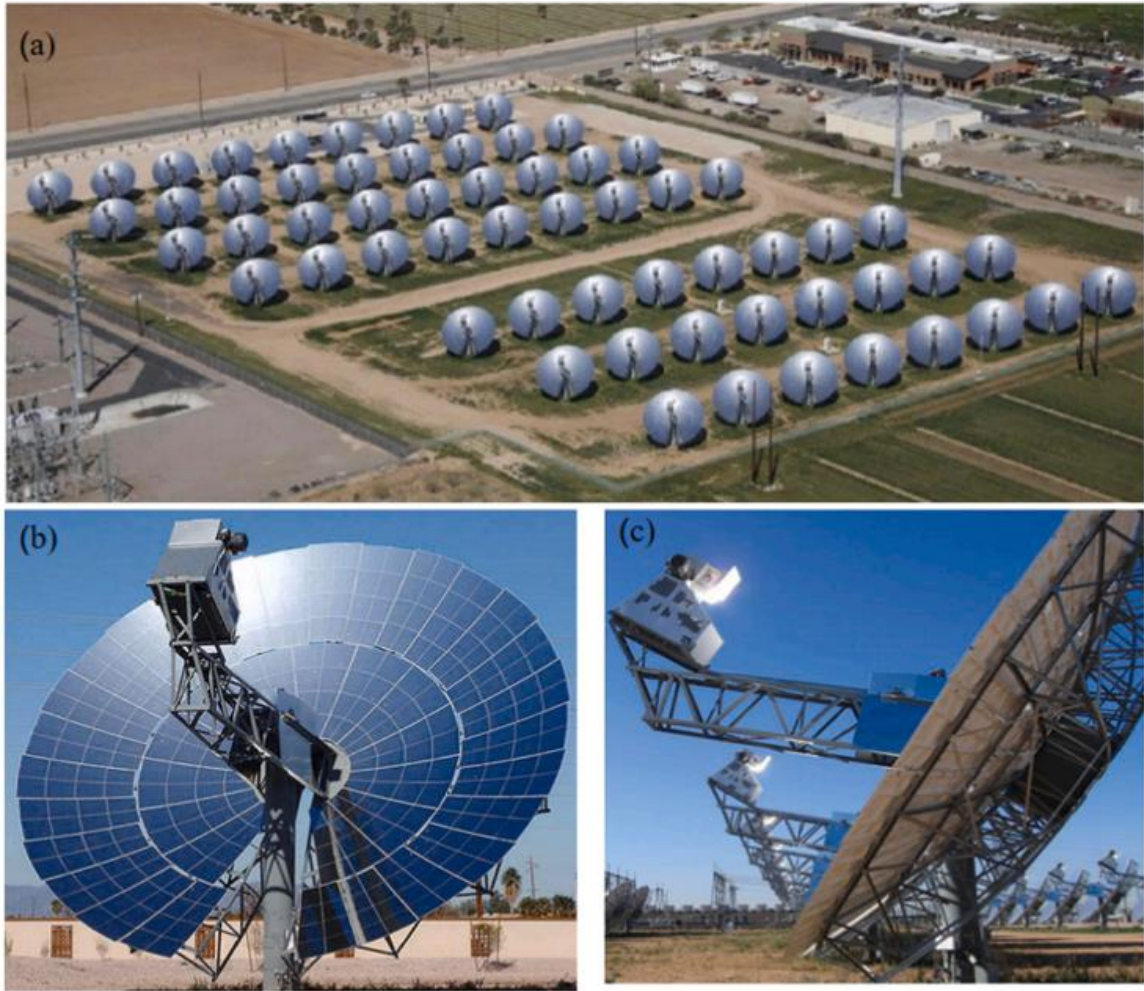
Figure 6: Fig. 1. (a) Maricopa SDSPP overview in Peoria, Arizona(Coventry & Andraka 2017) (b) Maricopa SDSPP unit-scale sun catchers SDSPP (Carrillo Caballero et al. 2017) (c) screenshot of Sun Catcher PCU (Ghodbane et al. 2020).
